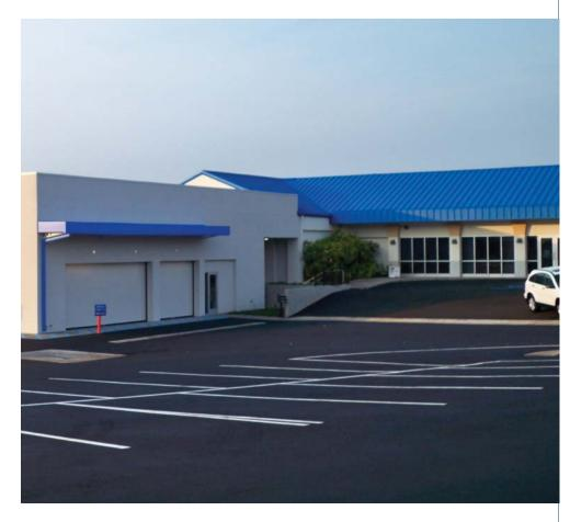
Renovation of existing parts boutique, parts storage, restrooms and showroom area. Construction of new Service Reception, Express Service Bay and Service Bay building. Work included demolition, site grading, site utilities, asphalt paving, concrete slab on grade, pre-engineered metal building, metal roofing, built-up roofing, roll-up doors, aluminum doors and storefront, drywall, EFS, acoustical ceiling, painting, ceramic tile, plumbing, air conditioning, fire sprinkler and electrical systems
