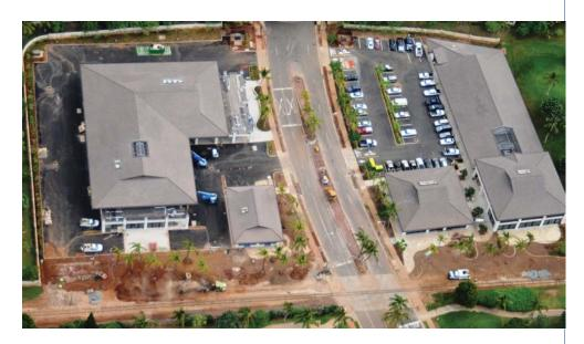
This upscale restaurant/retail/office complex at the Ko Olina Resort is a combination of cast in place concrete, structural steel and DEFS/Stucco shell with concrete tile roof and coral wainscoting.
